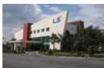
LSCV(HO Chi Minh) MV / LV cable UTP, Optical cable Overhead cable
