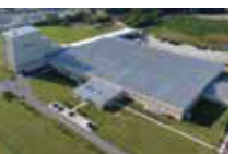
LSCUS(Tarboro) MV / LV cable Control, Instrument cable
